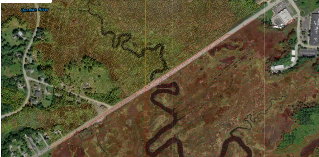
A section of Route 1 that can potentially flood in severe storms.
